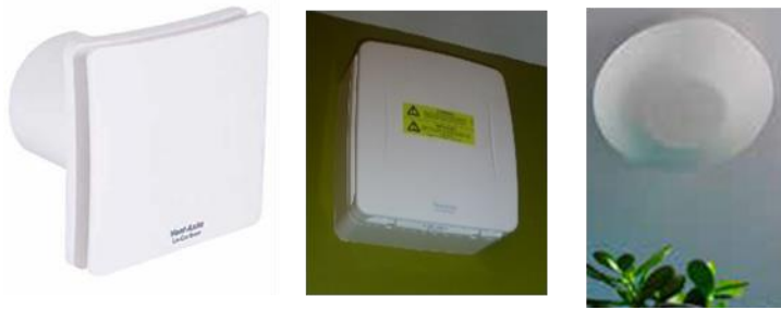
Figure 4.10 Images of mechanical extract fan included in the survey
