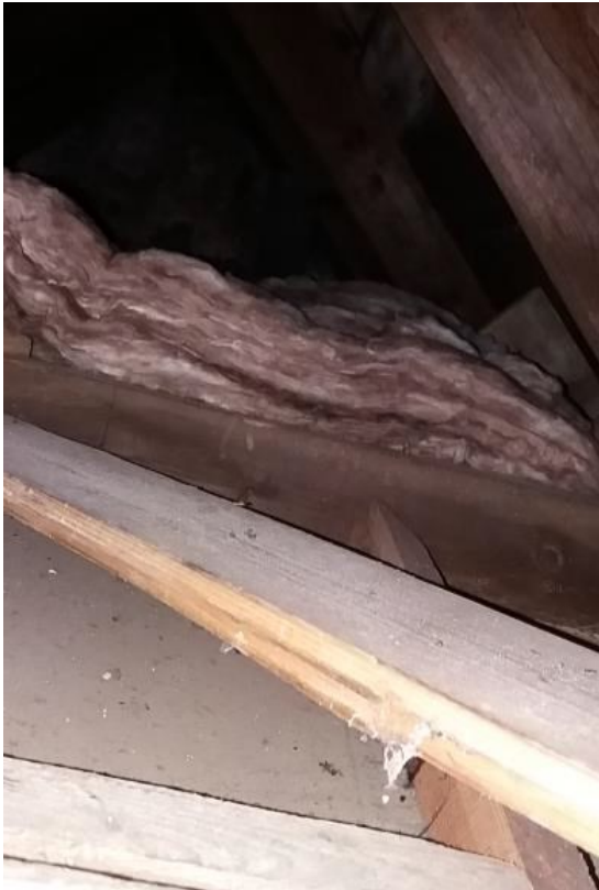
Photo 1: Loft space with some insulation
