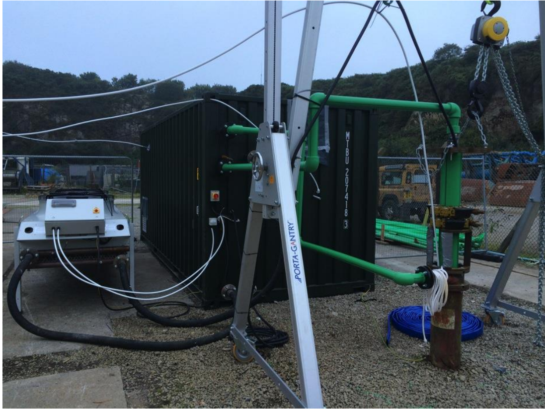
Figure 17 Thermal Response Test unit and connected energy abstraction fans
