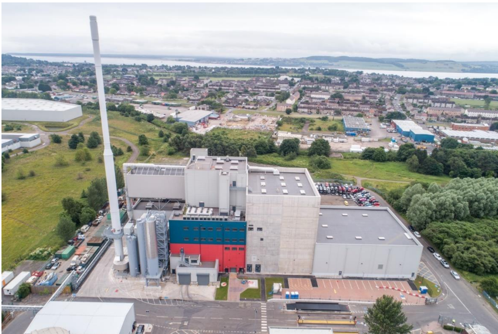
Figure 29. Baldovie EfW facility (Credit: MVV)
