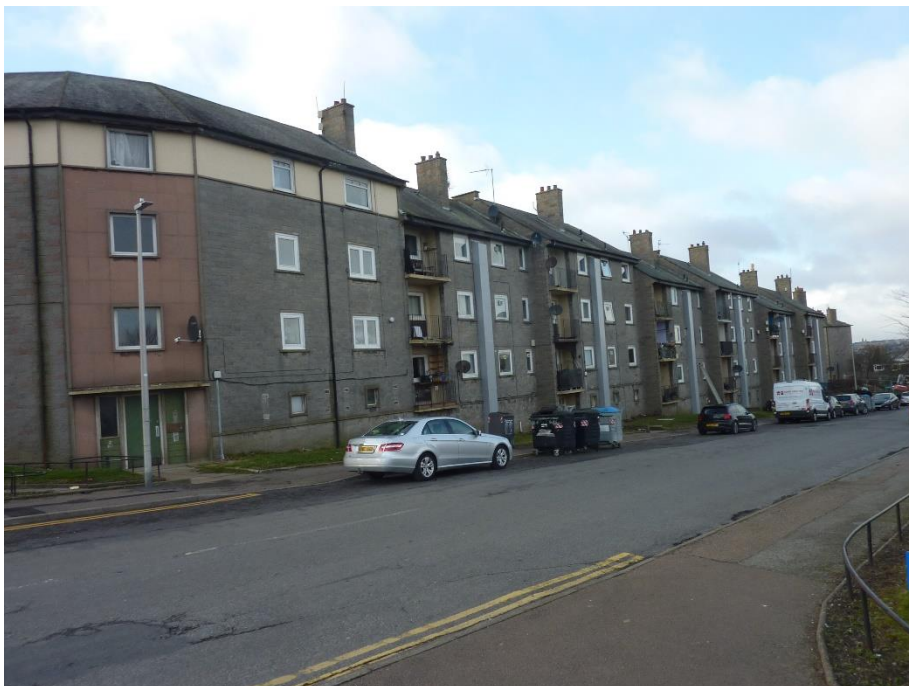
Figure 7. Domestic properties connected to the Torry Heat Network (© Aberdeen City Council)
