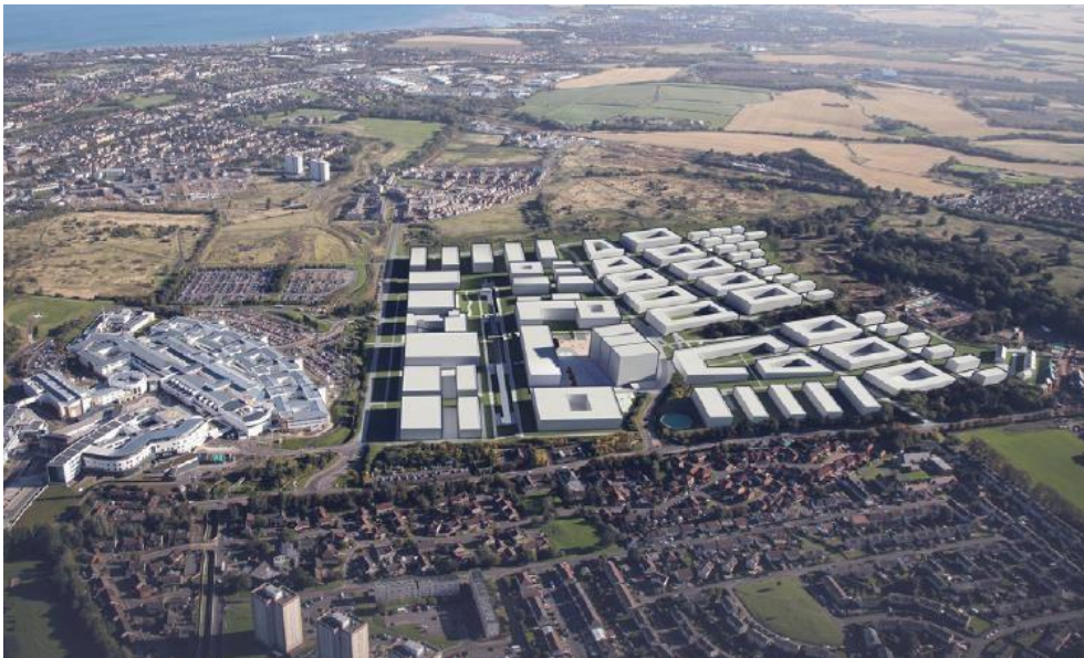
Figure 13. Aerial view of the Edinburgh BioQuarter site (Credit: Oberlanders Architects)
