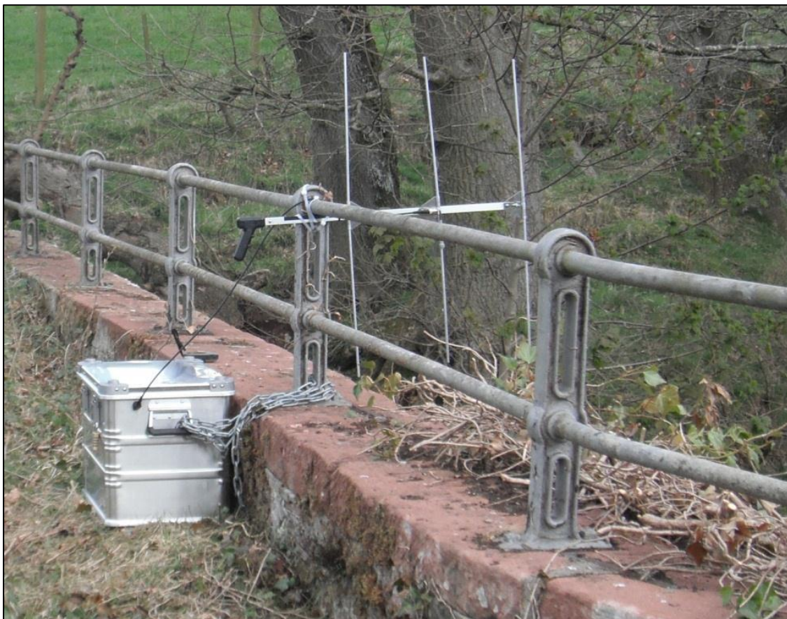
Figure 2.2.1.5: A typical fixed receiver station in situ . Note the watertight metal container which housed a rechargeable battery connected to a combined radio receiver / data logger box, in turn connected to an external radio antenna. This particular fixed receiver station was located at Shielhill Bridge (see Figure 2.2.1.6), a disused road bridge across the River South Esk. The installation is positioned high and directly above the river with the antenna pointing directly downstream, reducing the risk of flooding while maximising antenna “line of sight”. The antenna was attached securely to the bridge railings to maximise stability.
