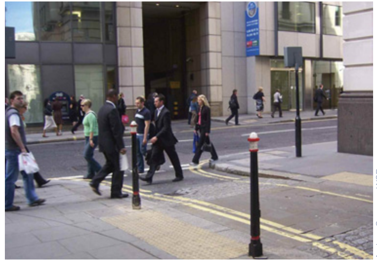
Raised crossover, but located away from the desire line for pedestrians and therefore ignored – the crossover should be nearer the junction with, in this case, a steeper ramp for vehicles entering the side street
