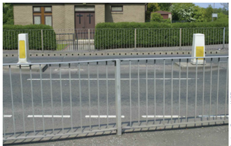
As well as being visually intrusive, the inappropriate use of guard railings can block pedestrian desire lines, with consequential possible dangers
