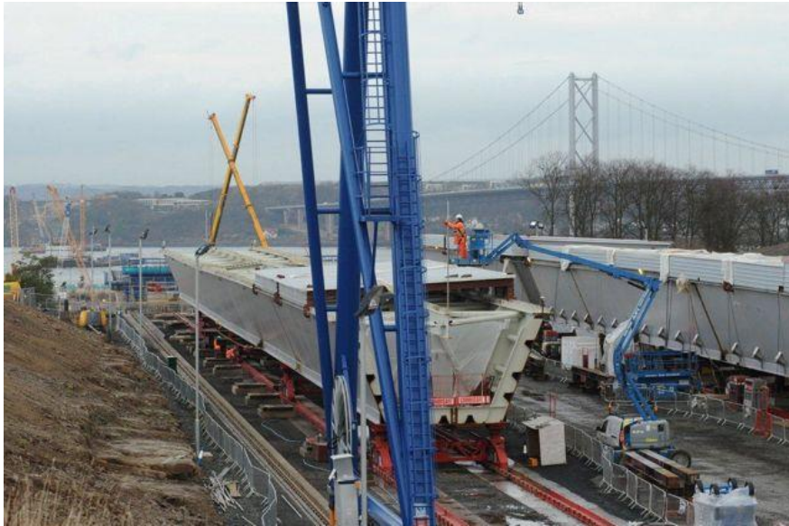
Construction of the Queensferry Crossing
