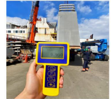
Proof of load test carried out on forward casing 0762 Port Side.
