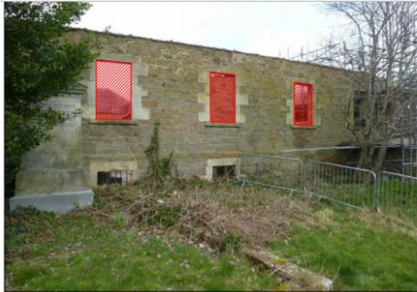
IMAGE OF CURRENT UNBLOCKED WINDOWS
